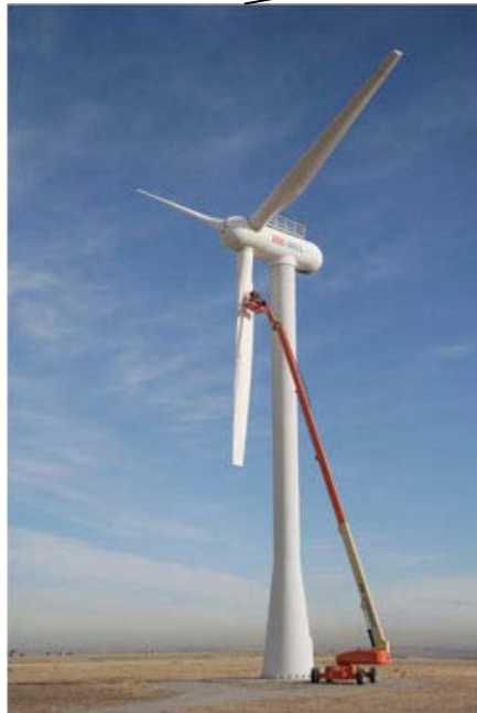
NREL CART 3 Closed-Loop Data Collection Source: nrel.gov/wind
