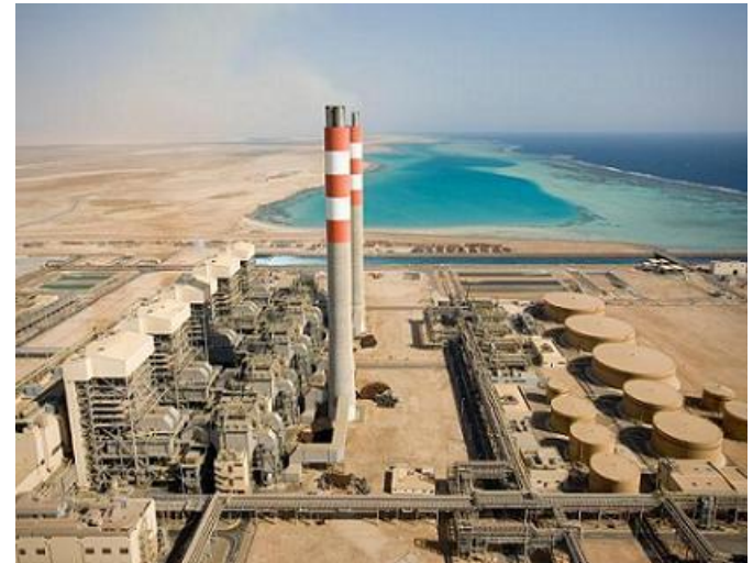
Shoaiba Power and Desalination Plant 3.6 million m 3 of water per day
